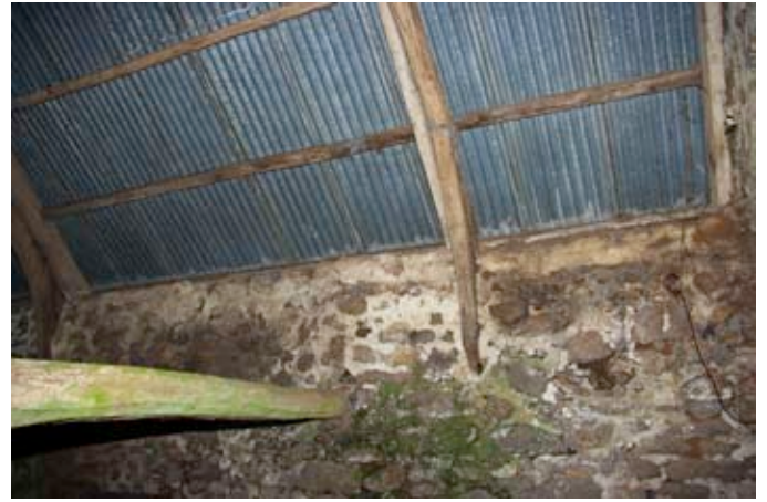
Inside the shippon nearest the current entry track.
